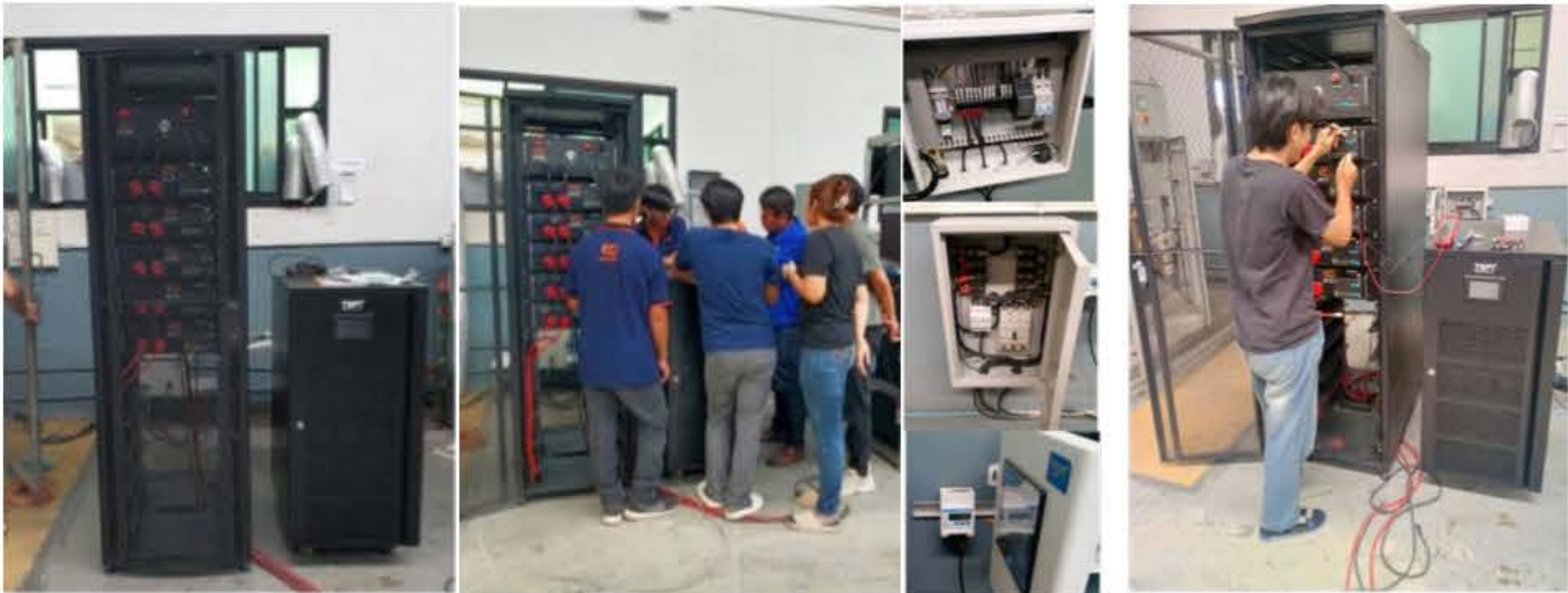
Figure 5. The connection between BESS, bi-directional inverter, and EMS.
