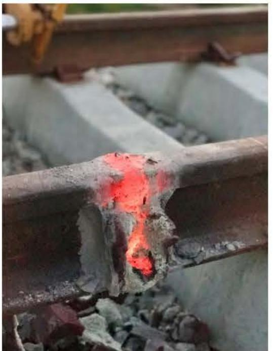
According to the measurements of thermite welding for rail steel grade R260, the welded hardness is 260-280 HB and the base rail hardness is 280-300 HB. Show that the welded has a lower hardness value than the hardness of the base rail.
